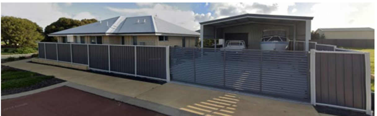
Google Maps street view of the existing garaport at 11 Twilight Drive, Jurien Bay
