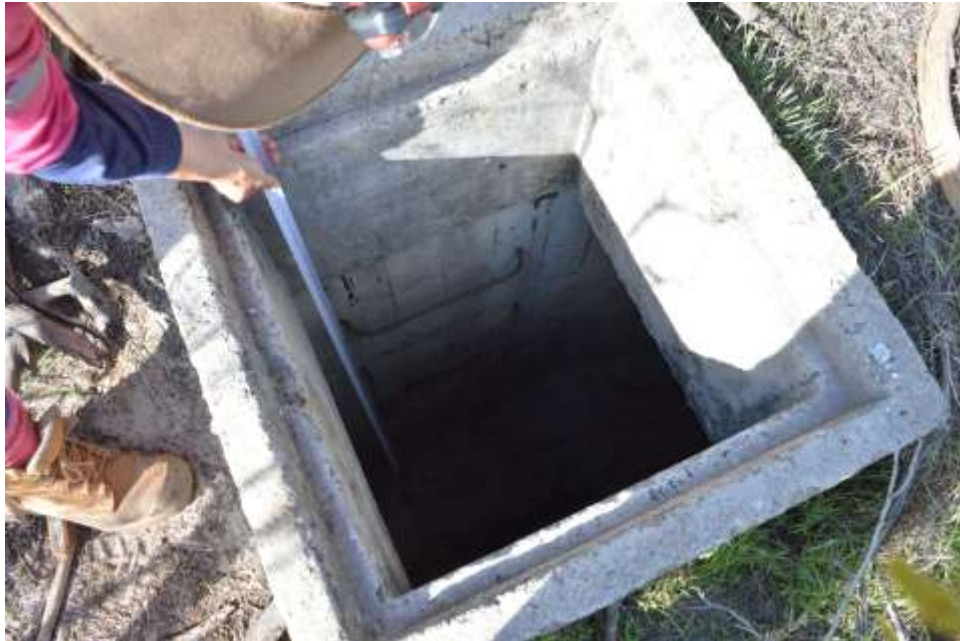
Figure 42. Cistern man hole. HDA photo.
